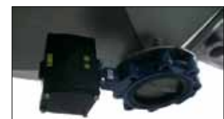
Automatic discharge valve
